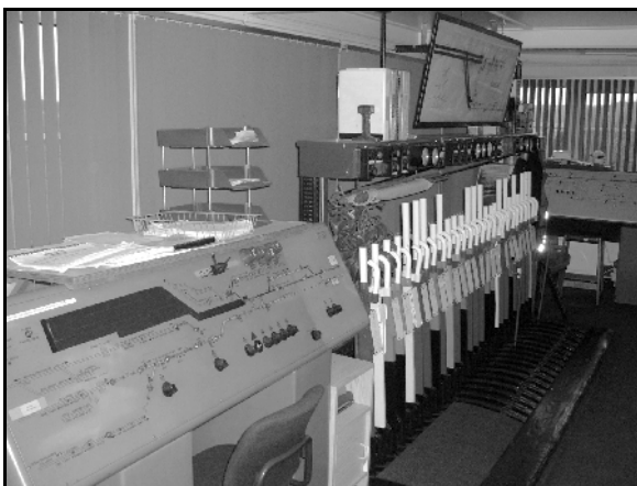
Clipstone West Junction box interior as seen on 22 nd Feb. 2006. The panel ex Concentration Sidings is on the left, with the remains of the lever frame beyond. At the far end is the NX panel which was installed after the closure of Welbeck Colliery Junction in 1997.
