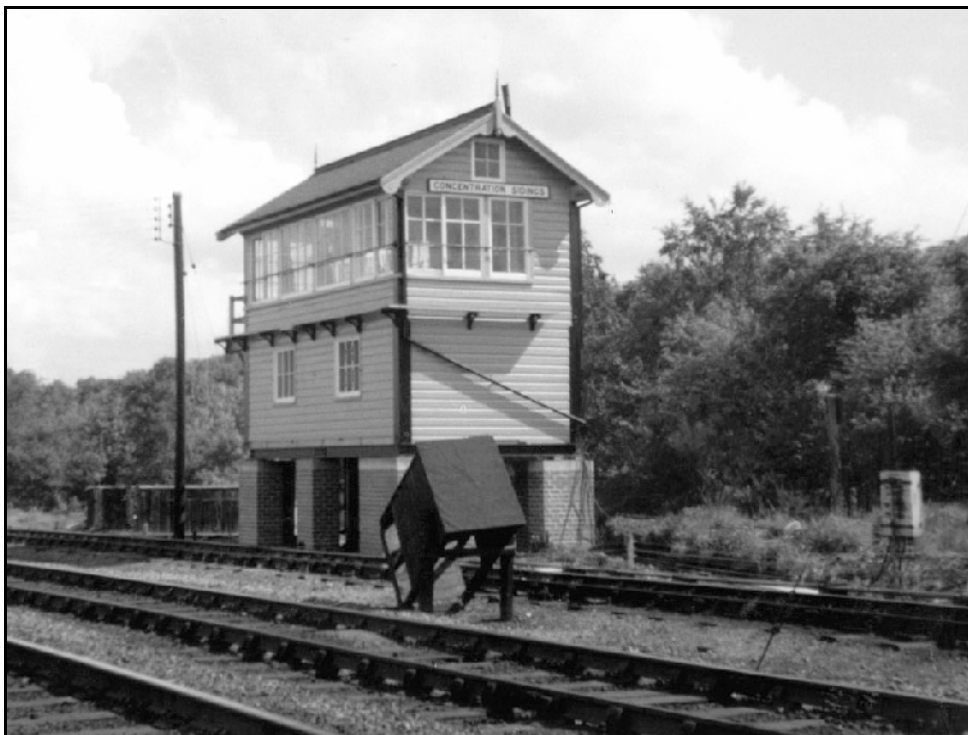
The GCR box at Concentration Sidings looking towards Clipstone Junction. It was originally built on wooden piles to allow an all-round view of the sidings, however as these rotted over the years, they were replaced by brick pillars. The wooden "shed" propped up is a fogman's hut. photo: Derek Talbot
